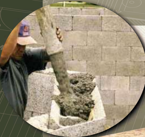
Pour concrete faster and easier without worries about blowouts, wall alignment or voids.
